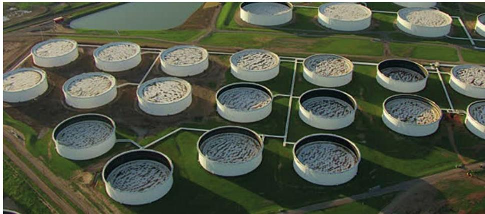
Maintaining high performing storage facilities can be challenging as paraffin and asphalt solids build continually over time, reducing effective tank volumes. Subsequent cleaning and the removal of tank based sludge deposits from your tanks can be a costly exercise. Down time for cleaning disrupts your cash flow and the cost of cleaning is often exacerbated by the increasing cost of hydrocarbon waste disposal and labour.
