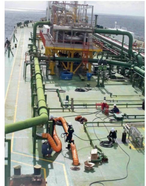
Work on the FSO was carried out above deck, administering HCD Tank Clean to the tanks below. Tank Clean successfully reliquefied sludge oil deposits in situ without the need for removal and disposal.
